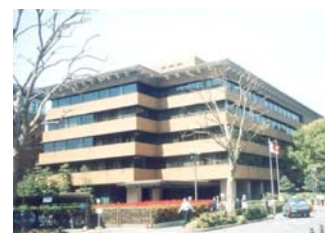
Assembly Building September 1975
