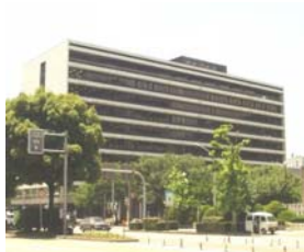
West Annex June 1964
