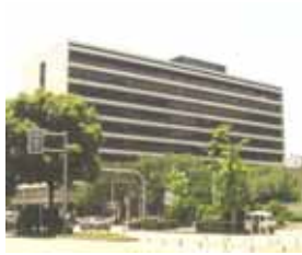
West Annex June 1964
