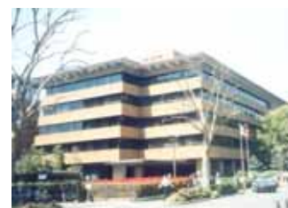
Assembly Building September 1975
