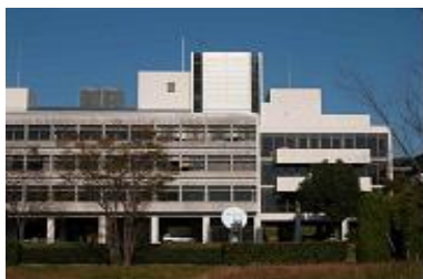
Exterior view of the Aichi Prefectural Education Center
