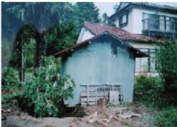
(b) 陥没穴と噴砂
