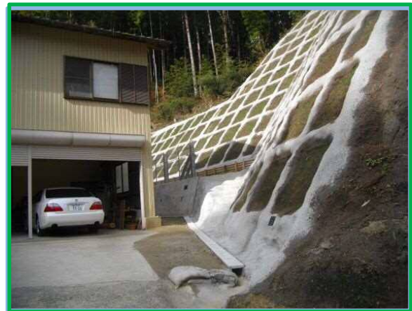
人家を守る治山工事
