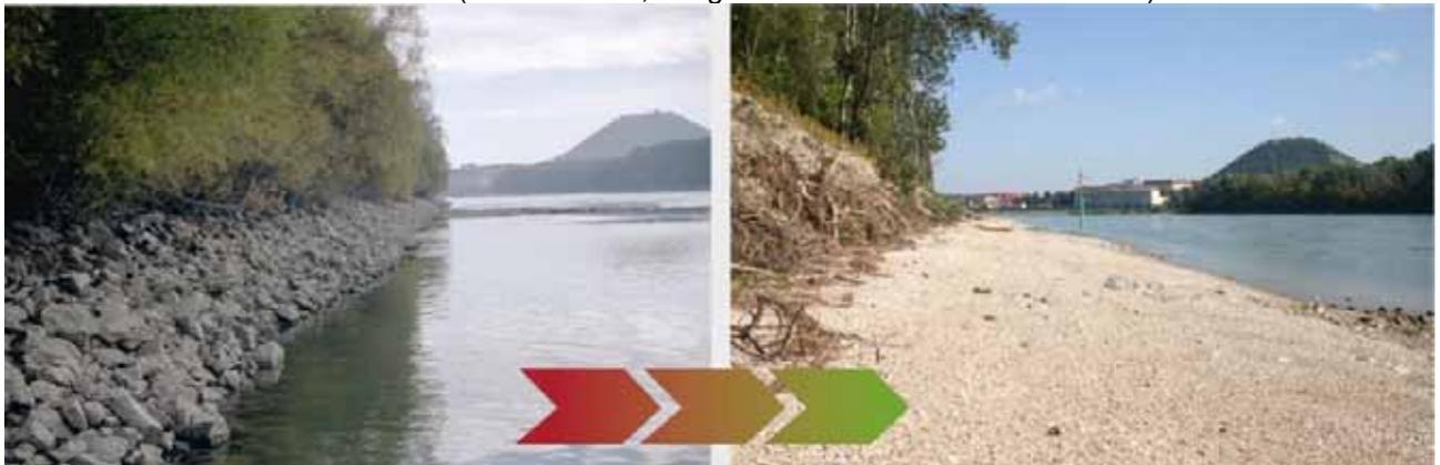
Down-sizing of groynes to improve ecology but without changing their effect for navigation: At left before the works; at right after intervention (at the same water level!): the groyne is now lower, oriented downstream and allows fish migration along the bank. © via donau
