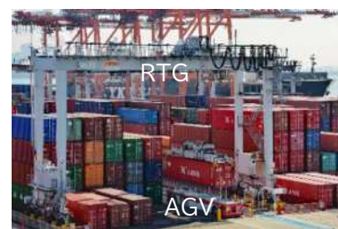
自働搬送台車(AGV)と遠隔自働 RTG
