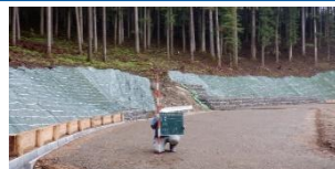
Paving of forest roads
