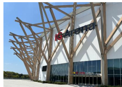
Construction of prefectural facilities
