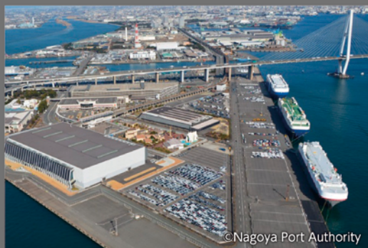
©Nagoya Port Authority
